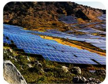
Mountain communication base station
