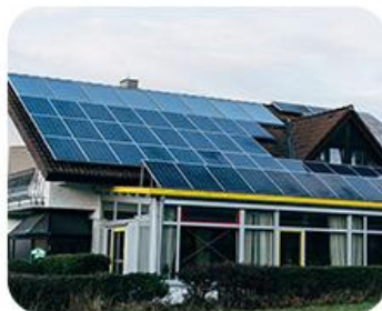
Home energy storage
