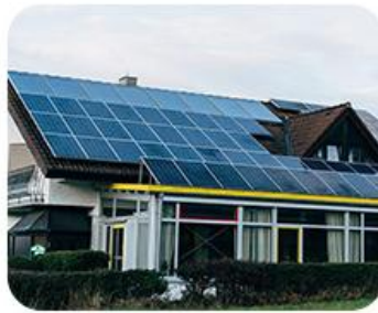
Home energy storage
